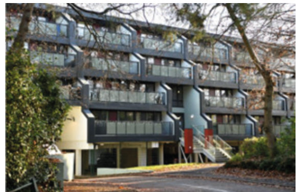
Balco's structural glass stairway balustrade
