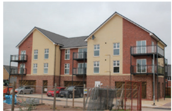
View of the site
